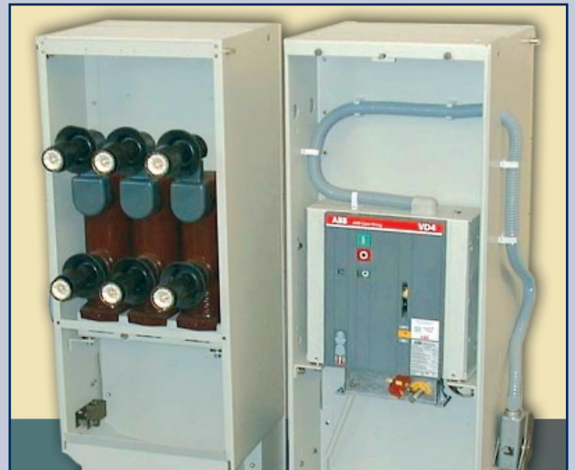
After retrofitting: 12 kV switch truck type ZE 5 with vacuum circuit breaker VD 4 .... 1250 A .... 31,5 kA
